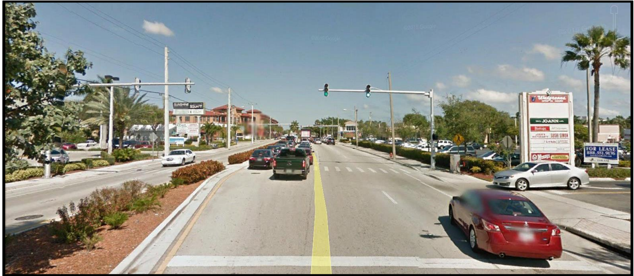
Figure 20 Photo of Federal Highway at location of Major Project Driveway
