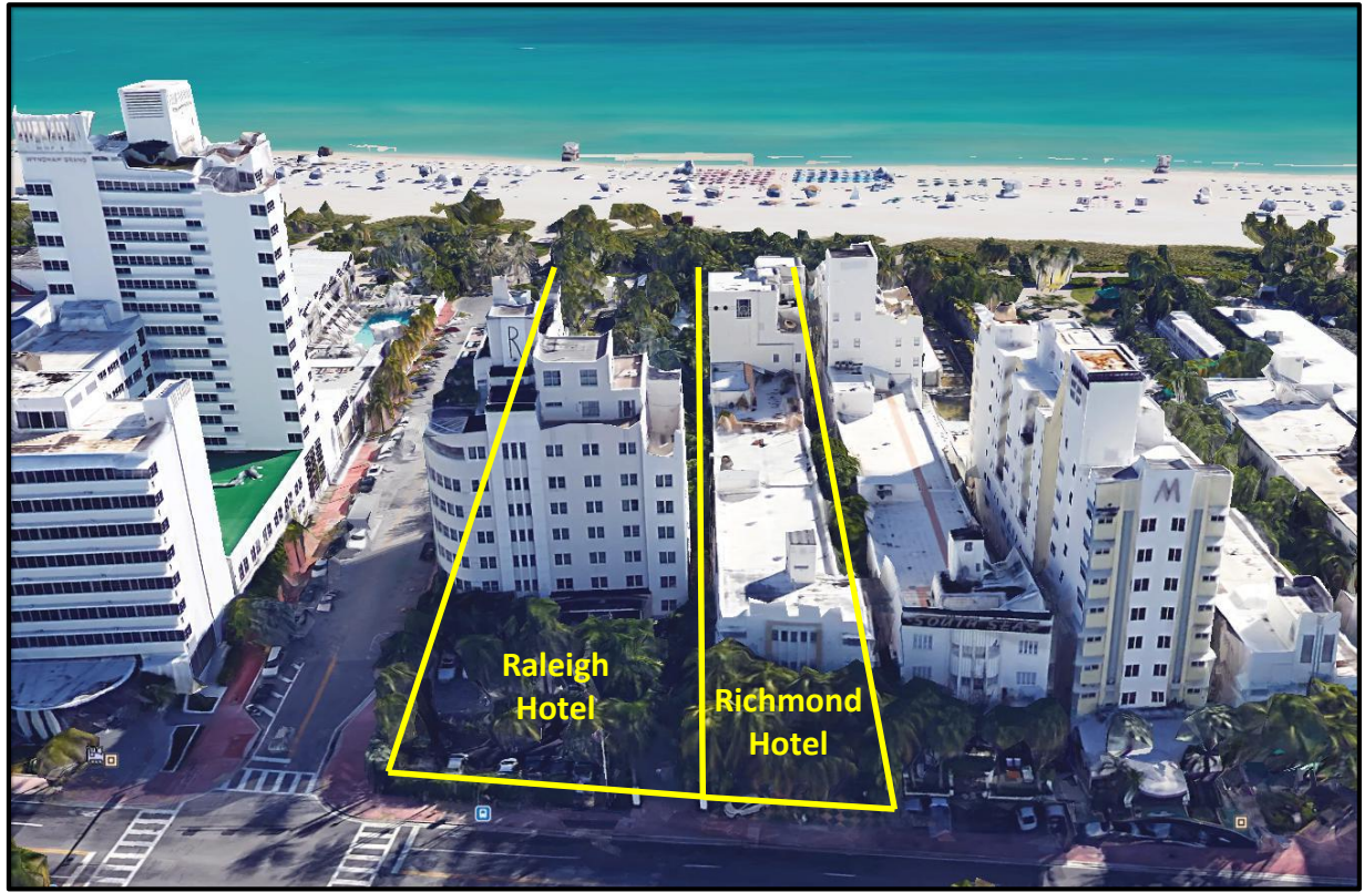
Figure 7: Oblique View from West with Property Highlighted
