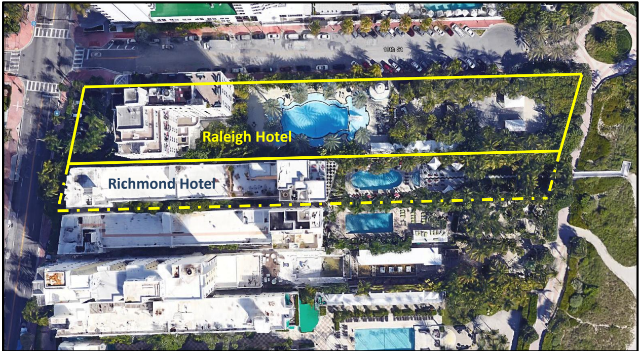
Figure 6: Aerial View of Raleigh and Richmond Properties Outlined in Yellow
