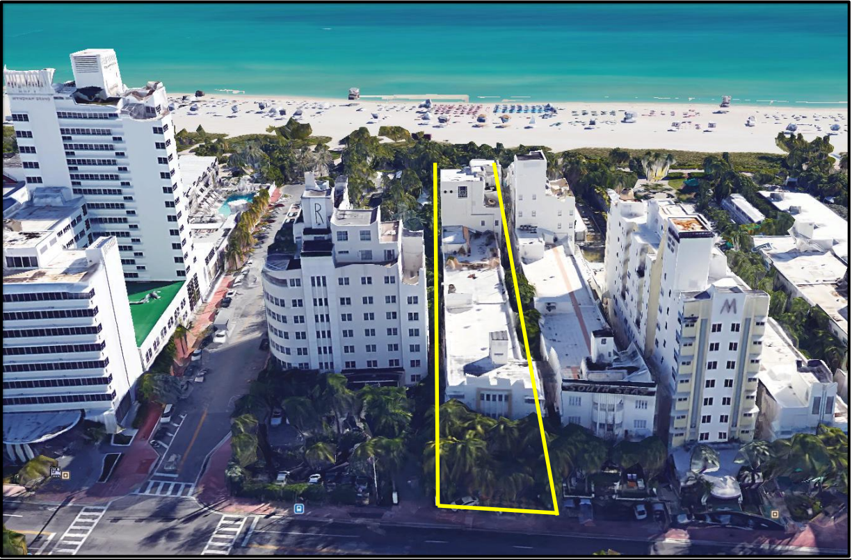
Figure 3: Oblique View from West with Property Highlighted
